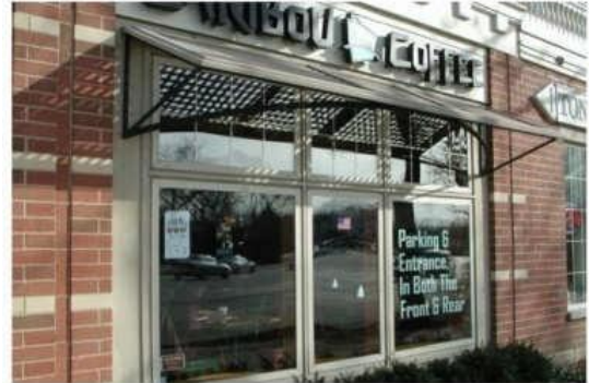
Permitted Awnings: Metal
