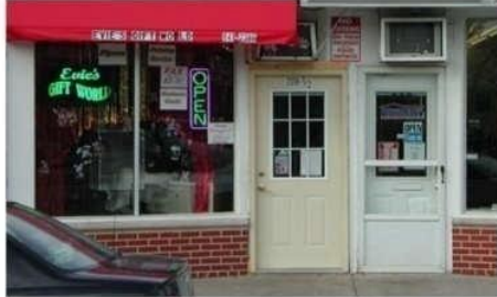
Prohibited: Residential Grade Doors on Commercial Buildings.
