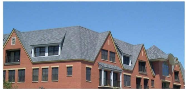
Roof Materials: Asphalt Composite Shingles
